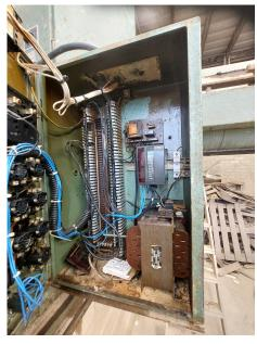
Control was via a run signal and a potentiometer, with a separate control for the home function. An aging control panel showing signs of modifications over the years had left the fast home function inoperable, this was rectified as a part of the project.
