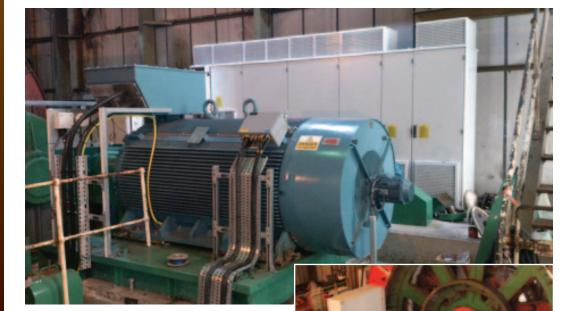
A 3.3kV to 690V LV drive conversion replaces an obsolete slip ring motor control system with a modern ABB ACS800 regenerative inverter, supply transformer and motor improving production and reliability at one of the UK's largest salt mines.
