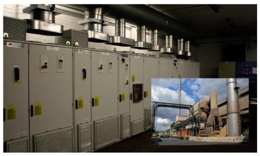
£650K 'Turnkey' Variable Speed Drive project replaces an existing troublesome 3.3kV DOL Extraction Fan Control System and saves over £200K+ in energy annual costs.
